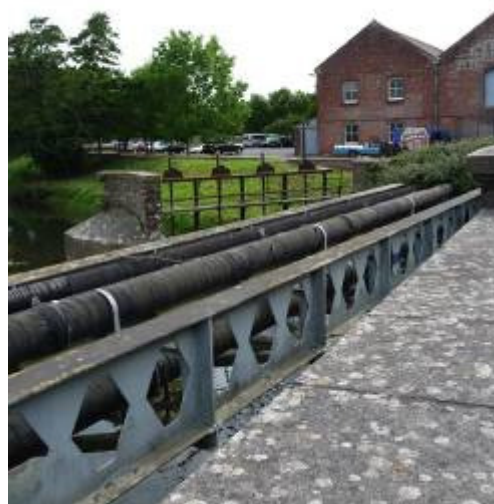
Figure 2: Site of Hatches and Service Pipes for nearby housing estate
