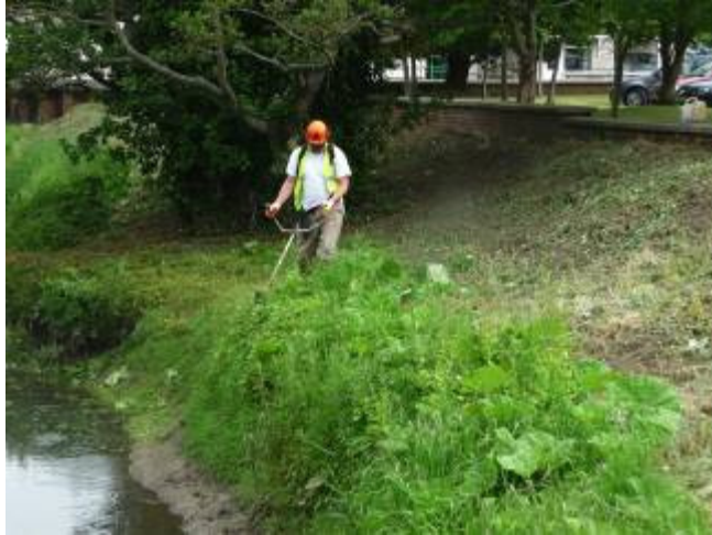
Figure 4: Strimming the bank to encourage Water Voles to move upstream prior to commencement of works as part of the recommendations from the Water Vole Survey
