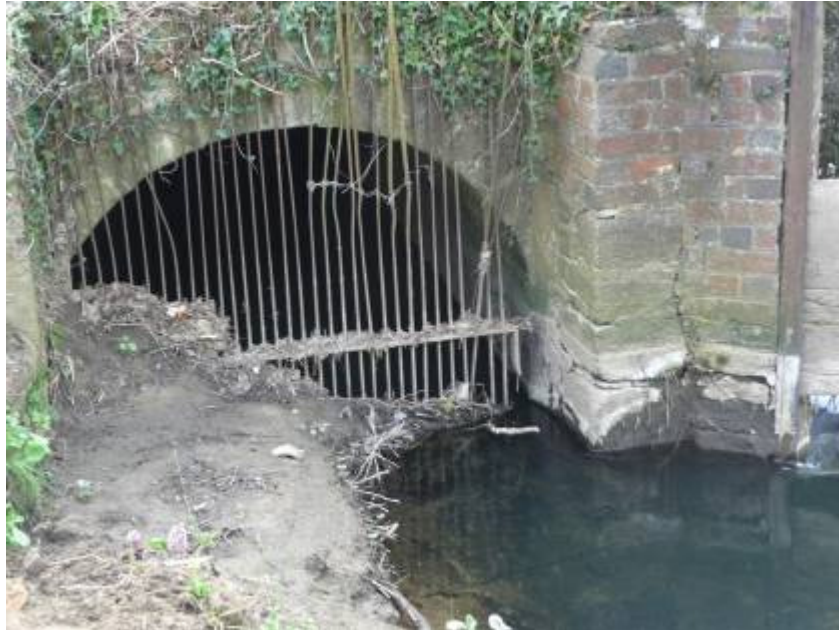
Figure 7: Leat used by Palmers to draw water to turn the water mill. Siltation in front of the leat has caused problems in the past and required manual removal.
