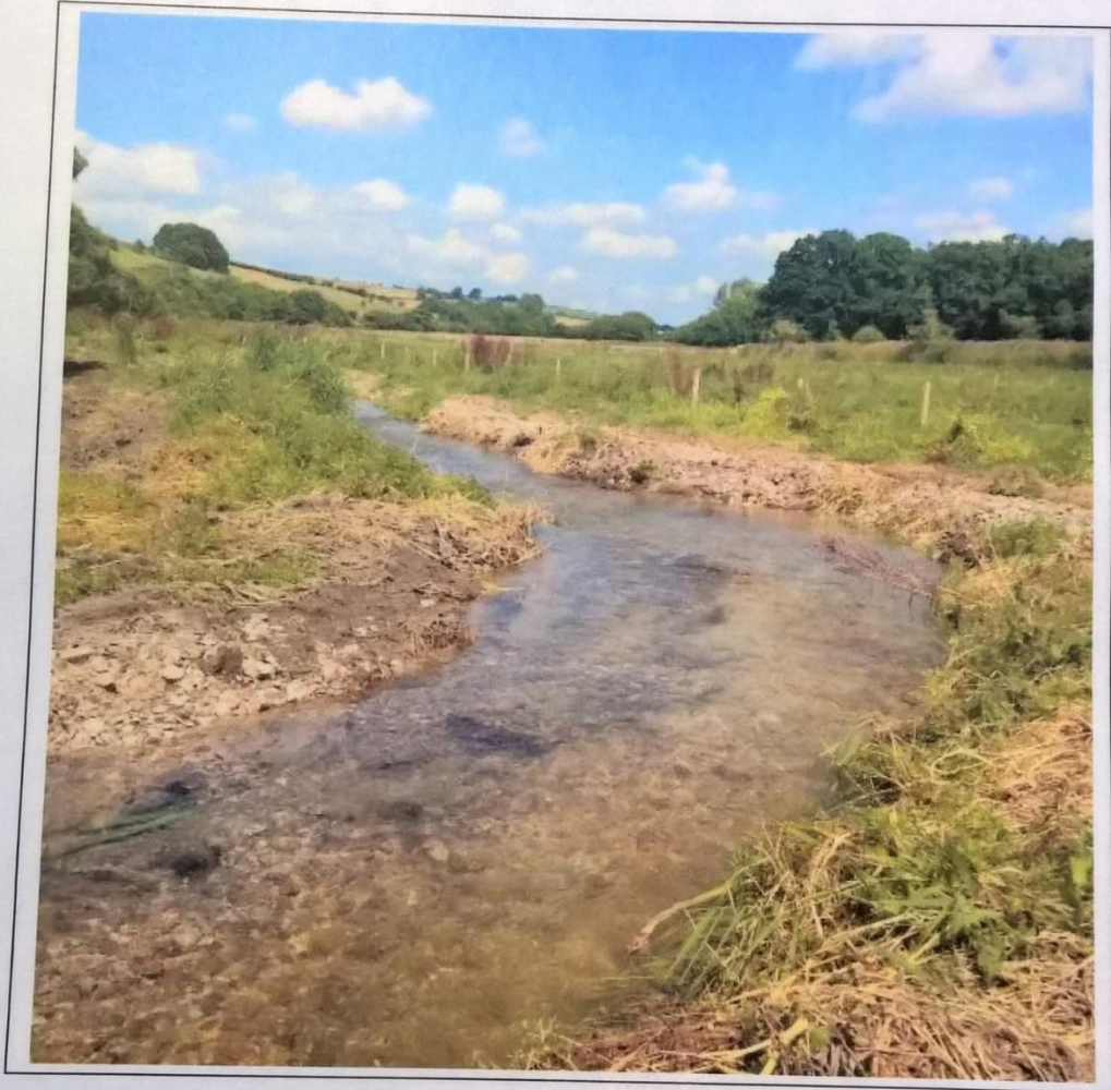
The Sydling Brook bypass channel following restoration work by Five Rivers Ltd
