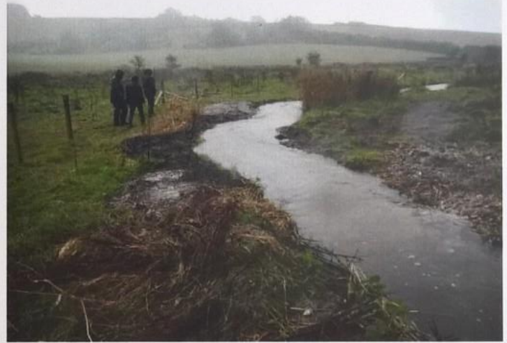
The Sydling Brook artisan fish pass, before (left) and a new meander in the bypass channel
